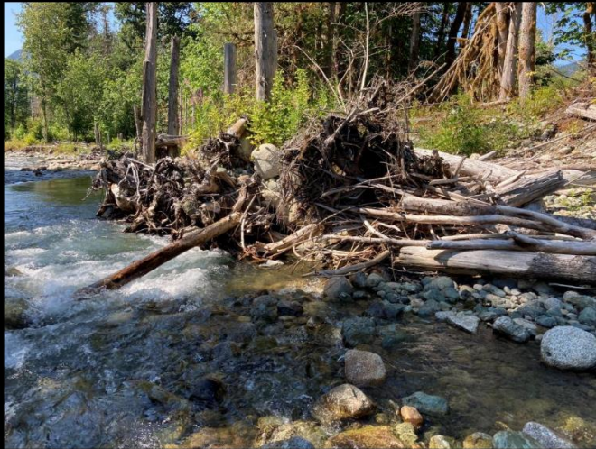
ELJ formed pool with wood accumulation, channel A, July 2021.
