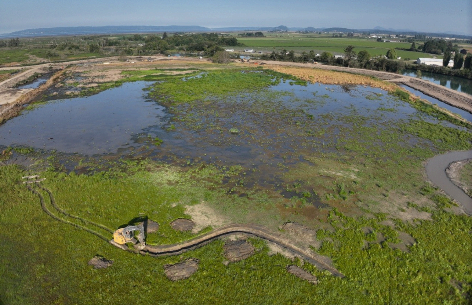
Photo: Constructing a tidal channel on the west island at Island Unit, August 7 th 2026. Provided by WDFW
